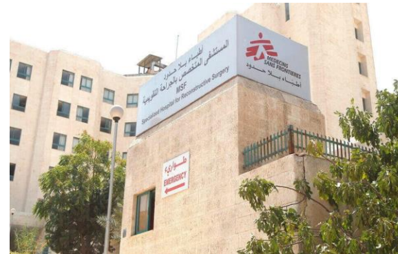
MSF Reconstructive project Amman (Jordan)
