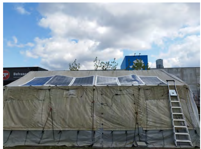
MSF is developing a solar energy rapid deployment kit that can be installed on the roof of tents commonly used in emergency responses, with the capacity to supply 9 kWh/day of electricity.
